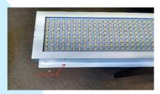
2. While holding the Brite Cor module to the desired surface, transfer the drilled hole locations to the drywall. Remove the Brite Cor Module and drill (4) 5/16" diameter holes.
